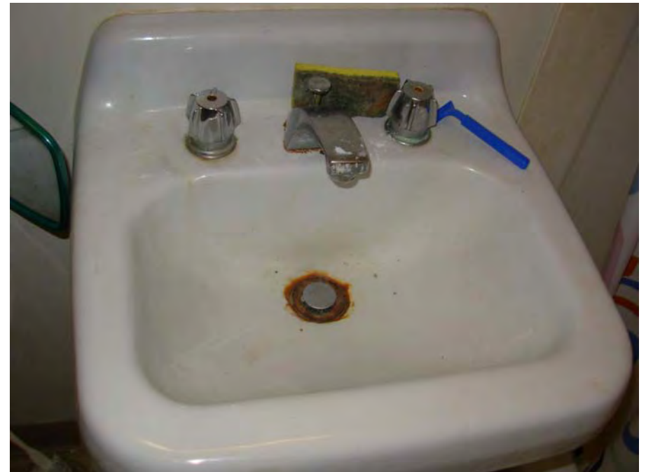
12. Some unit bathroom sinks with rusting at drains
